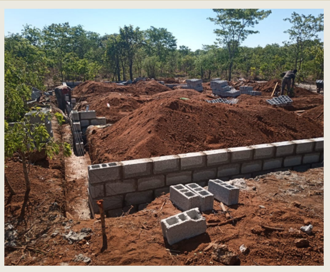
The beginning of the Wildlife Rescue offices
