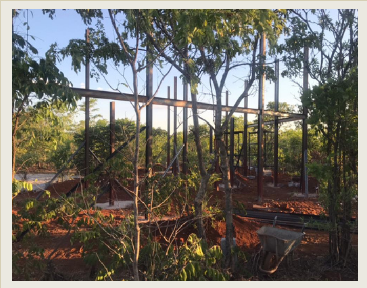
The steel structure of the elephant viewing hide
