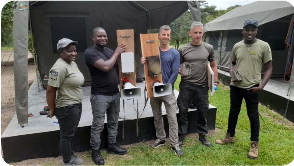
The GRI – Hack the Planet Team, ready to install the elephant repeller system
